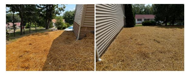
As well, they've disconnected the downspouts from the underground thing and they now discharge to the surface. I didn't see splash blocks under them, but they could have been hidden under the straw. If there are none, then I recommend going to Lowe's or similar and getting some plastic splash blocks and putting under the down spout outlets.
